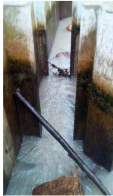
Fig. 6a, b, c: Fishpass at the Rosegg-St Jakob power station/ St Martin weir, blockages due to the entry of woody debris. © Sabine Käfer
